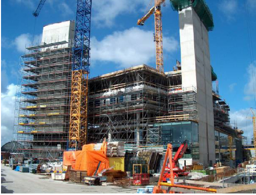
Figure 10. The library under construction.
